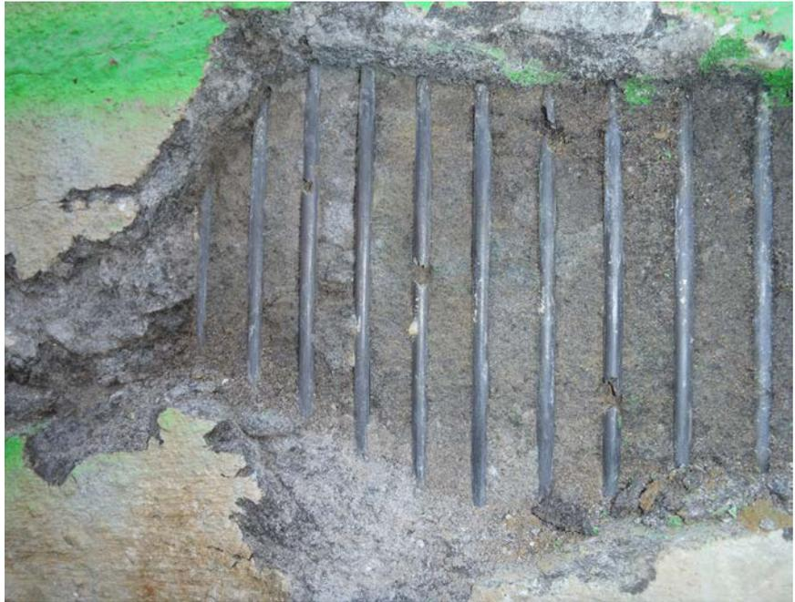
Broken wires on a PCCP main can be seen in this photo.
