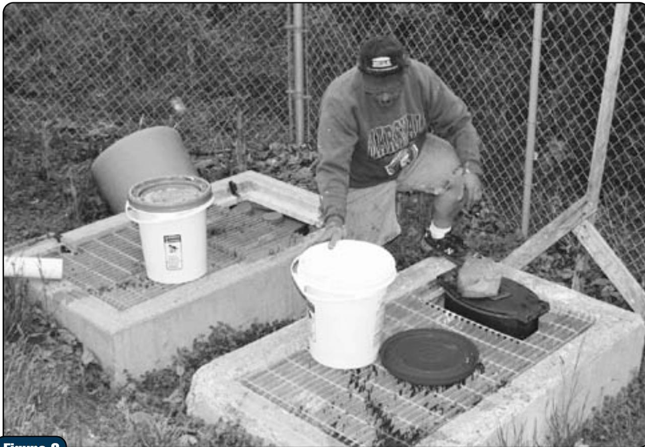
**Figure 3** At this package treatment plant, the wastewater is sent to the chlorinator then to the dechlorinator before final dispersal. [Please note that operator should wear gloves when handling chlorine tablets.] Photo by Chris Metzgar, NESCA.
