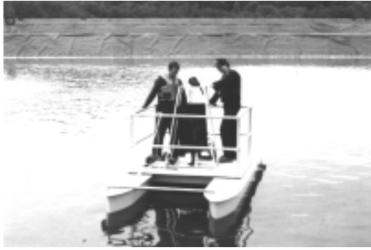
Jeff Saucier (left), superintendent of the Mars Hill, Maine, wastewater treatment plant, and John Peavey, operator, ride on a pontoon boat to inspect and clean the aerators in the lagoon system after five years of operation. (Photo courtesy of Jeff Saucier.)
