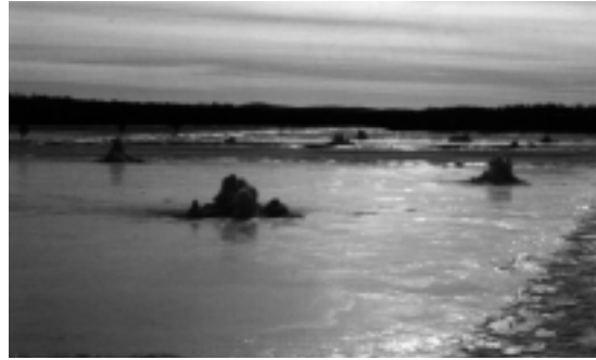
Ice towers in the Mars Hill treatment lagoon formed during the winter of 1998-99. The air tends to keep a small hole in the ice above the aerators where bubbles are formed and freeze. The bubbles pile up and form a volcano-like structure with a hollow core. These bubbles only tend to form on days with low atmospheric pressure, according to Jeff Saucier, plant superintendent. (Photo courtesy of Jeff Saucier.)
