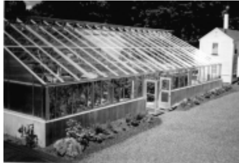
This greenhouse facility treats the wastewater for the downtown commercial center of Weston, MA, to groundwater recharge standards (tertiary treatment). (Photo courtesy of Ecological Engineering Associates, Weston, MA.)
