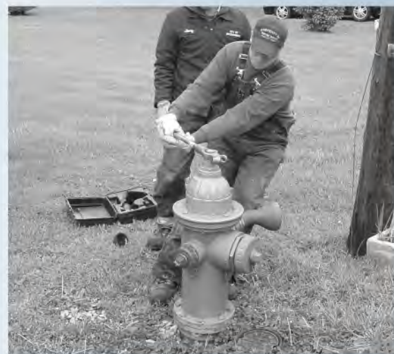
3. When finished, make sure to turn the hydrant securely off.
