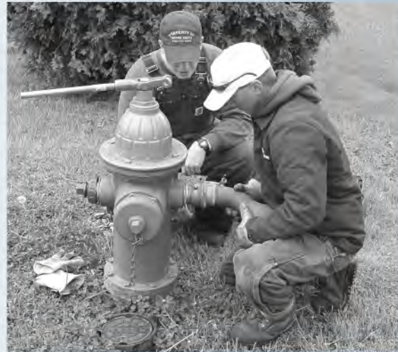
1. Flushing distribution lines is a two-person job.
