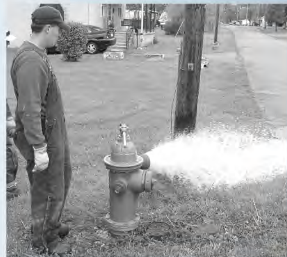
2. A diffuser protects property.
