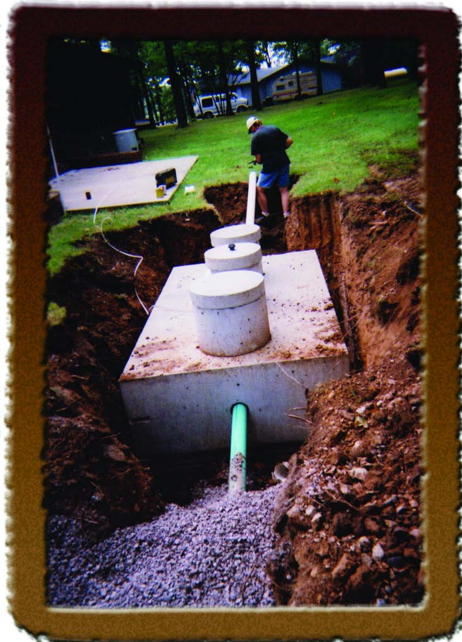
New septic systems are banned at Indian Point, Missouri, to be replaced by advanced treatment units, such as this aerobic treatment unit with biokenetic filter. Lateral lines (above) feed from the treatment unit (right). A distribution box (pg. 36 bottom and pg. 37) sends the lines to the filters (pg. 36 top).
