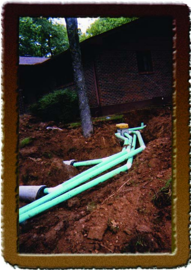
New septic systems are banned at Indian Point, Missouri, to be replaced by advanced treatment units, such as this aerobic treatment unit with biokenetic filter. Lateral lines (above) feed from the treatment unit (right). A distribution box (pg. 36 bottom and pg. 37) sends the lines to the filters (pg. 36 top).
