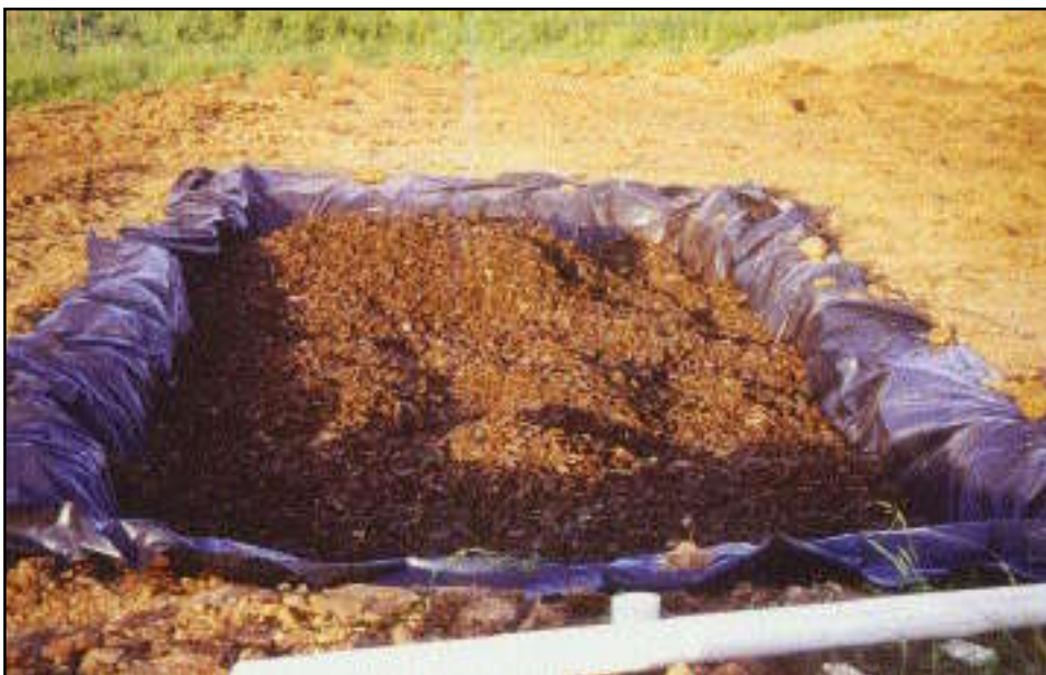
A subsurface-flow constructed wetland cell in Iowa uses tire chips as aggregate. Photo by Bill Milani.
